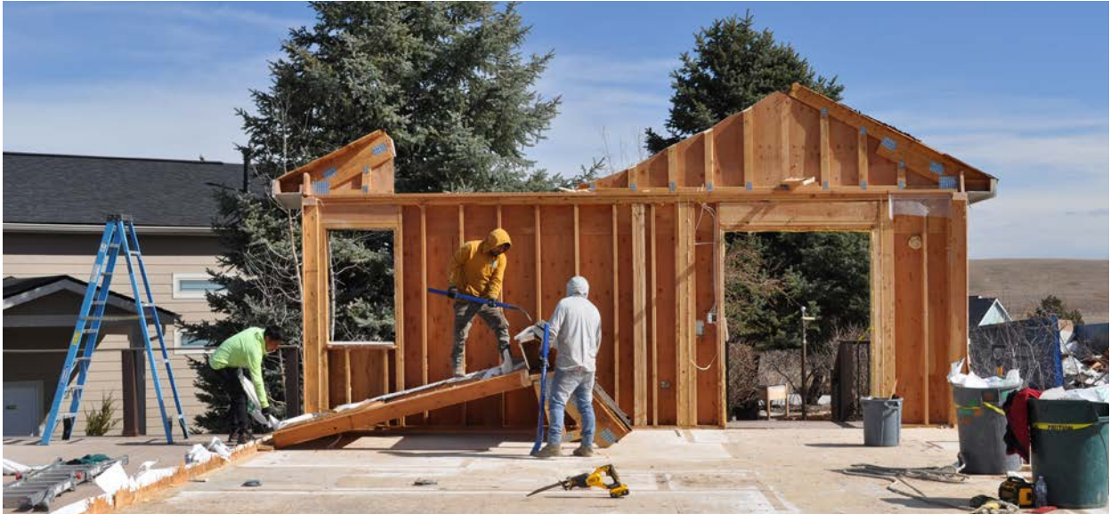
Deconstruction project by Perks Deconstruction, a nationally recognized leader in deconstruction based in Commerce City, Colorado
